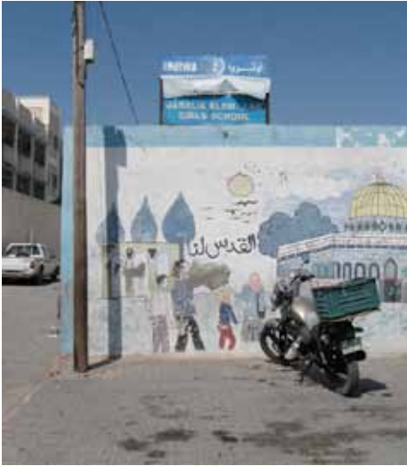
Damaged UNRWA shelter, Jabalia Elementary Girls School, north Gaza. Photo by OO, 19 Aug 2014
